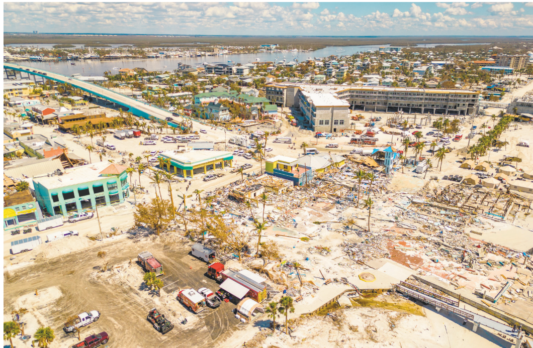
Massive destruction on Fort Myers Beach after Hurricane Ian.
